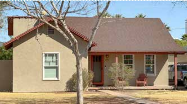
This homeowner replaced their wood windows with new ones that are the same size, material, and have the same number and configuration of panes in the upper and lower sashes.
